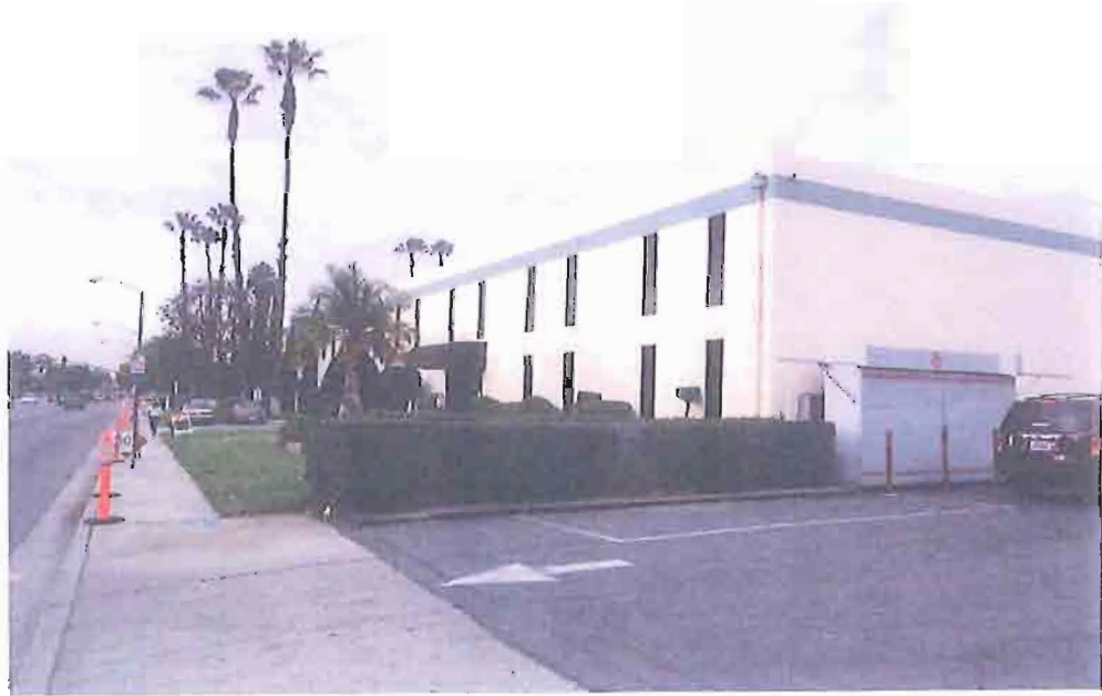
3- VIEW FROM SITE TO THE WEST
